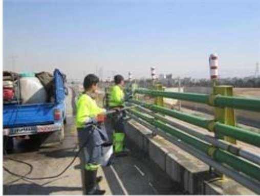
Fig.1. Traditional method of guardrail cleaning[2]
