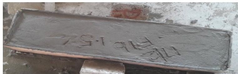
Figure 3 Reinforced beam casting
