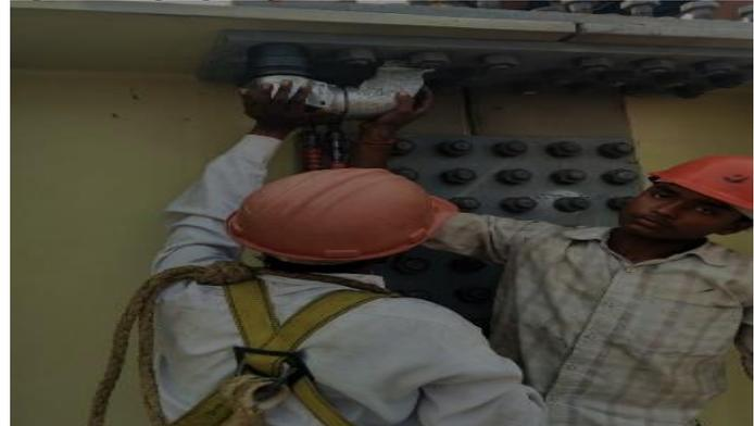
**Fig.2:** Bolt and torque adjustment
