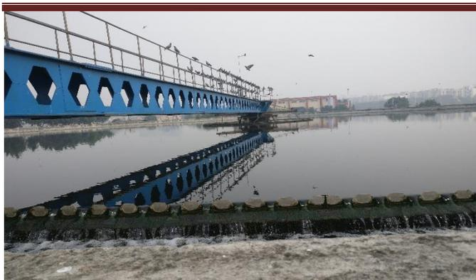
**Fig.7:** Secondary Clarifier of Okhla Plant
