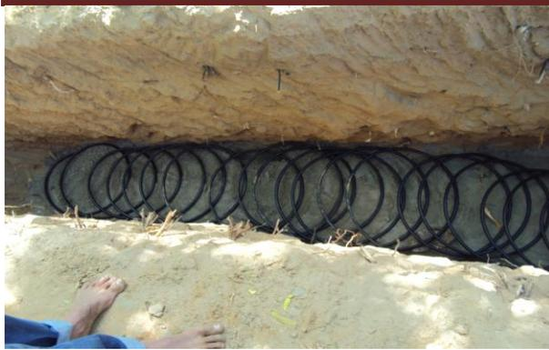
Fig: 2. Coiled form of the Pipe used in the Setup
