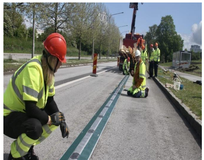
Fig: Construction of the electric roads (E-Roads)
