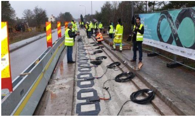
Fig:9 Development of inductive charging on roads
